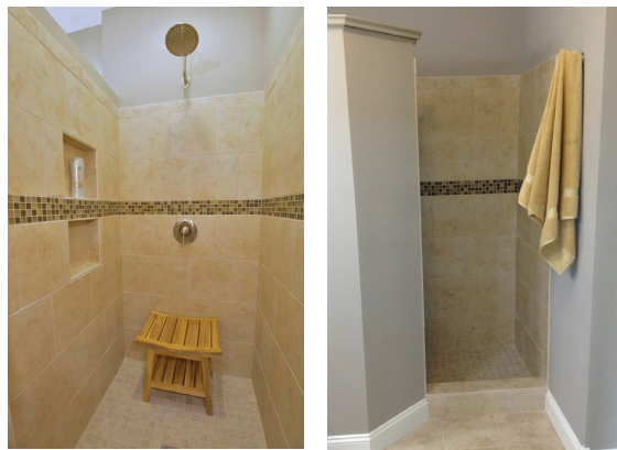
Shown with staggered tile. Composite white crown molding installed on exterior wall.
